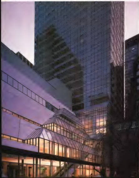
Doubling space without flexing muscles: Architect Pelli's garden escalator hall, with tower
